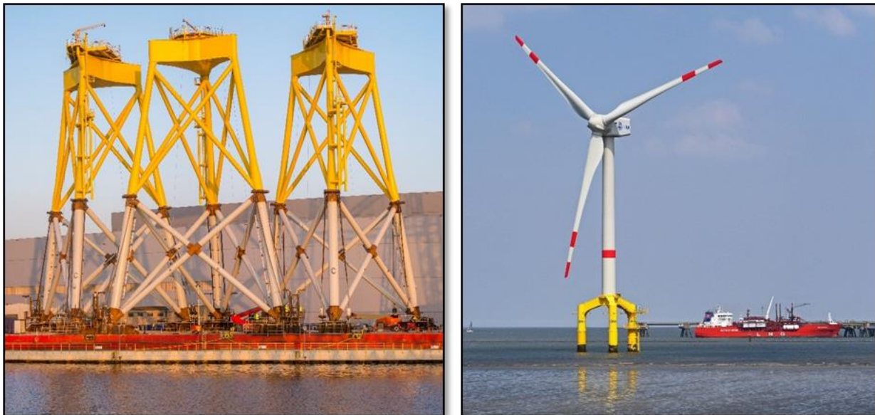
Figure 2-15. Jacket foundation (left); Triple foundation supporting an OWT (right). Source: Mike Marren (left) and Erich Westendarp (right).
