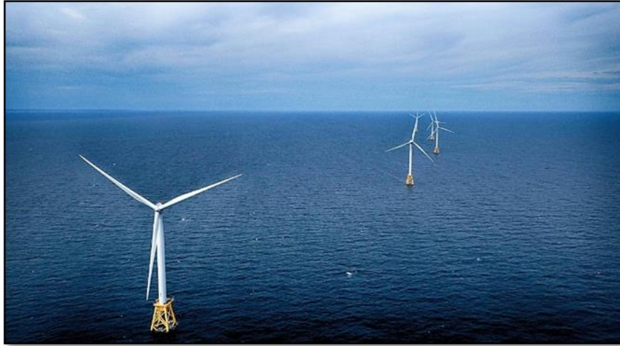
Figure 2-6. Linear arrangement of an OWF, the distance between the turbines is clearer than in the horizontal view.
